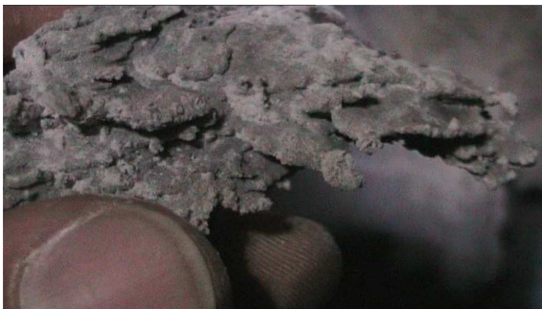
Figure 160. Crumbly brittle rock, close up
