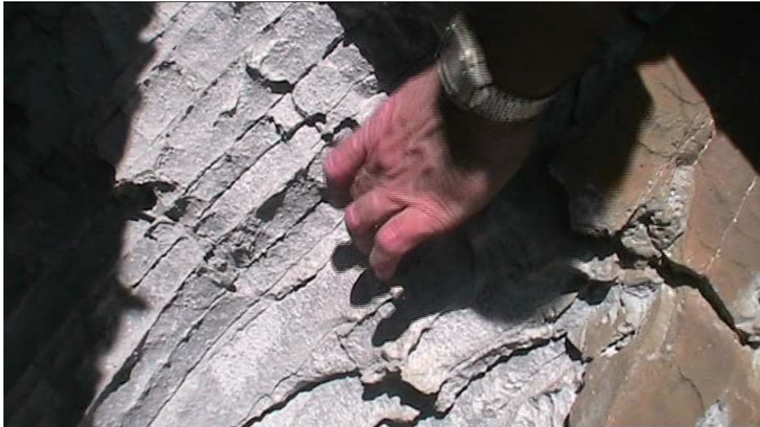
Figure 167. Outside the upper mouth of the Mank Master cave - Rapidly eroding soft powdery rock, decaying behind a surface of brown mineralisation
