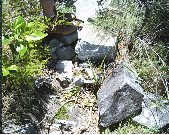
Figure 98. Fallen Pillar, East face
